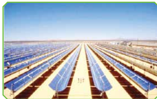
Parabolic Trough Power Plant
