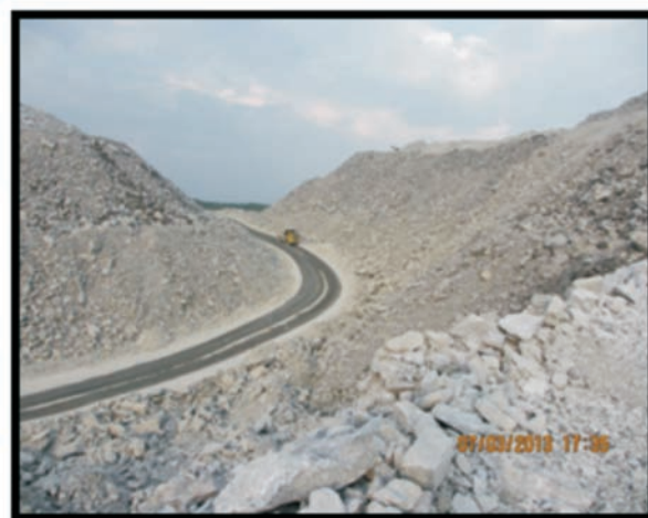
Huge rock debris
