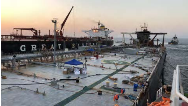
Figure 9. The unique over-the-top STS operation in progress
