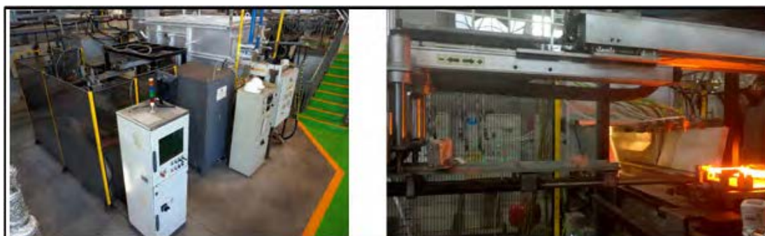
Figure 4: RINA descaling experimental facility
