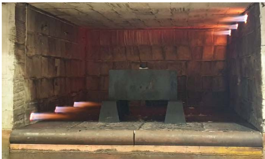
Figure 6:Image of the FAV industrial furnace during the test run with the six burners working
